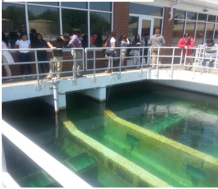
8 th Grade Trip-Blue Planet Water Treatment Center
